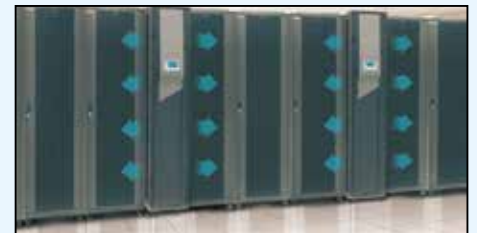
Figure 4: In-row cooling
