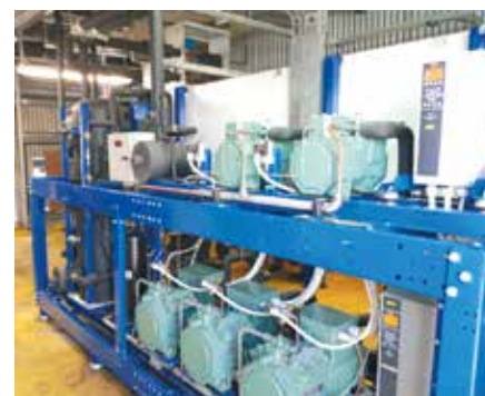
The CO 2 Transcritical Refrigeration Rack
