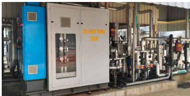
Figure 2: R744 Industrial heat pump chiller unit. 120 kW hot water production, lifting from 27^{\circ}\text{C} to 90^{\circ}\text{C} . Chilled water 12^{\circ}\text{C} to 7^{\circ}\text{C} .
